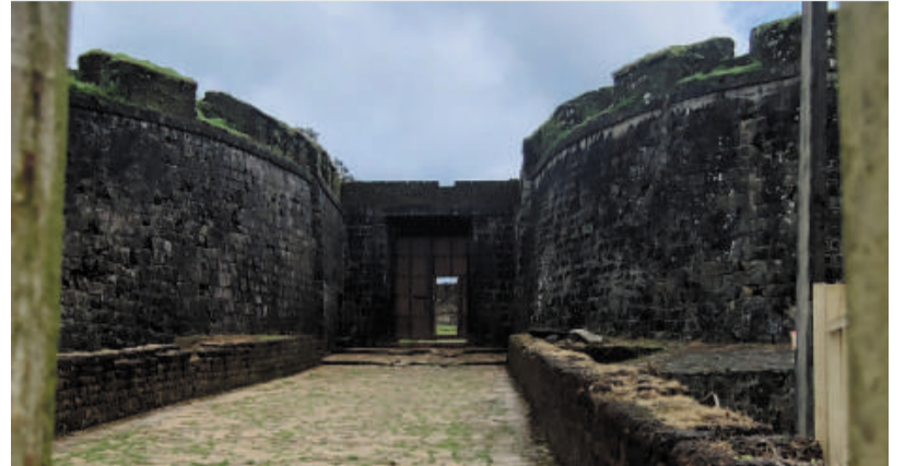
Entrance of Nagara Fort.
