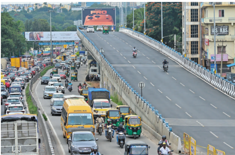
New 700m Hebbal Flyover Loop
